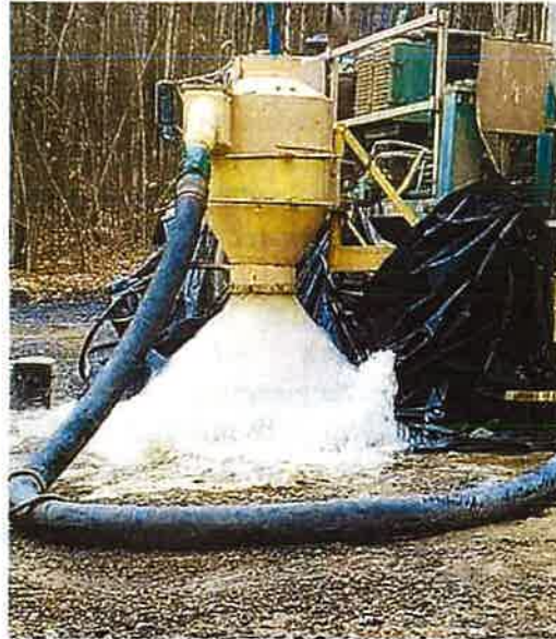
Very high rate of water production from cyclone on drill rig during well installation
