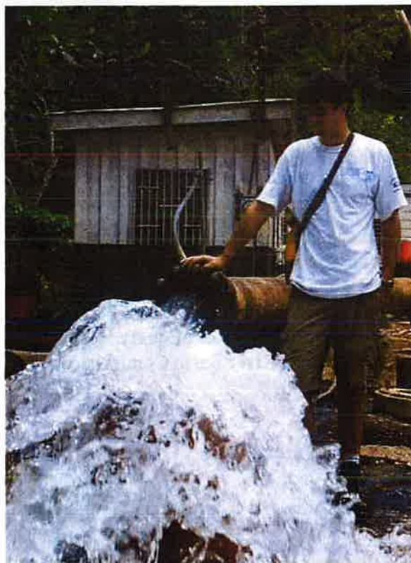
1,000+ gpm discharge from one of several similar yielding wells HSA sited and developed for the Water and Sewerage Authority of Trinidad and Tobago
