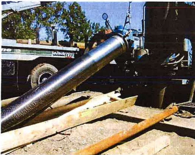
Installing 20-inch diameter screen in new production well for the Houghton-Caneadea Water District
